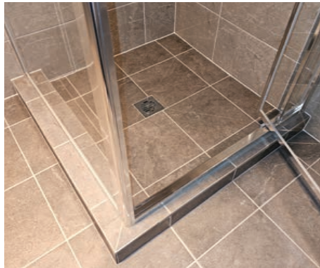
Shower Hob Construction
