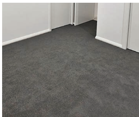
Carpet to First Floor, Stairs, Bedrooms and remainder of home
