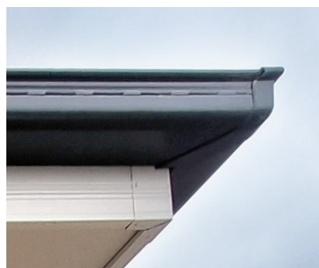
Metal Fascia & Gutter
