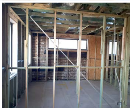
90mm H2 Timber Treated Frames
